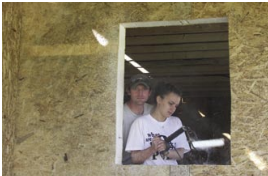
SIPS window cut-out for dog houses.
