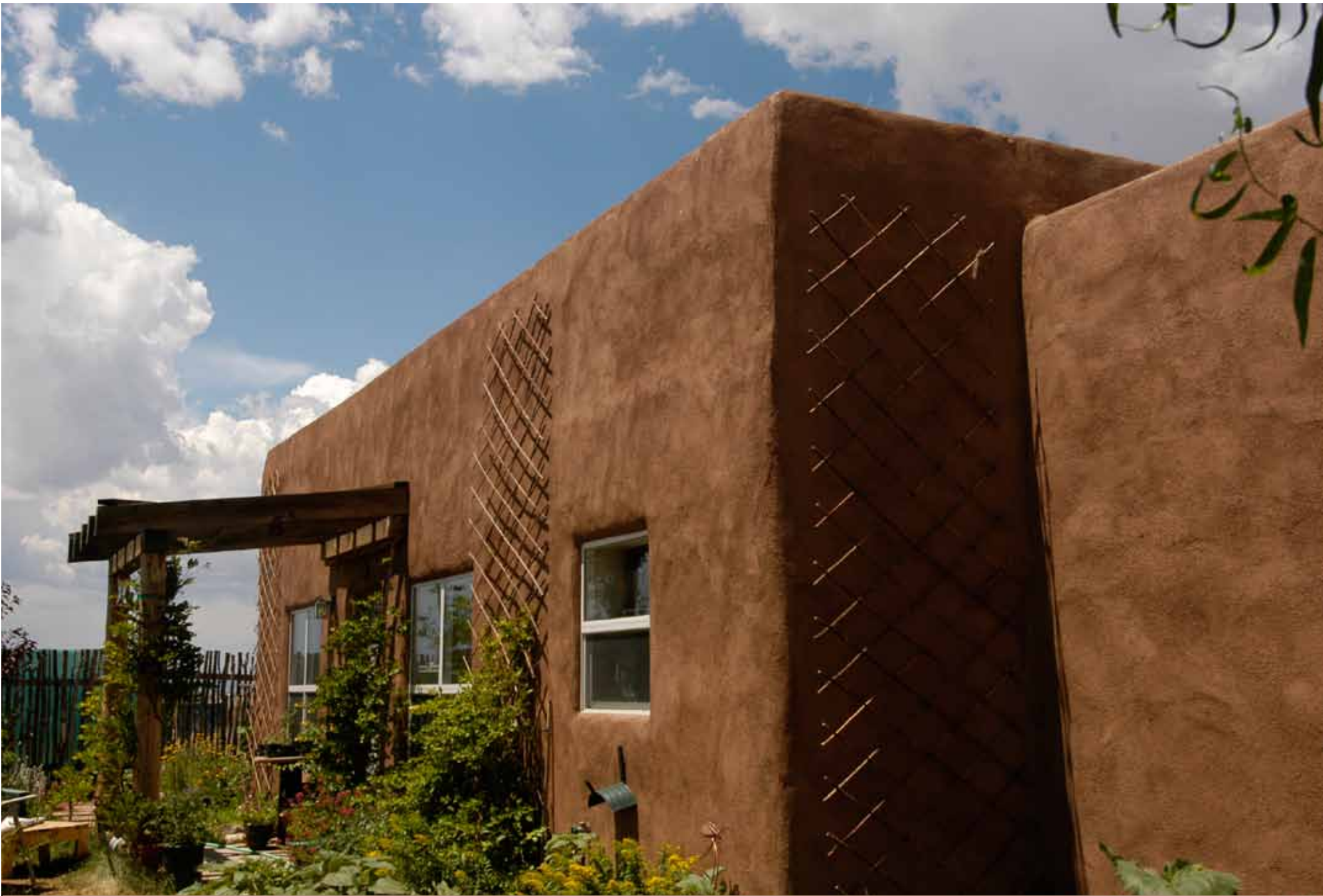
An adobe house in Taos, N.M., built with Habitat for Humanity in 2006.
