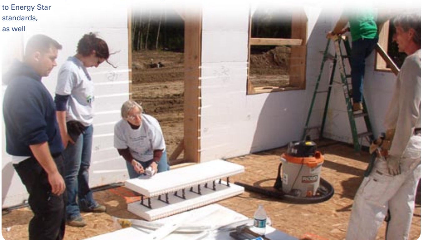
ICF CONSTRUCTION COURTESY OF HFH SOUTH PUGET SOUND
