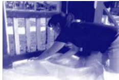
Cover the floor with plastic and seal it with duct tape.
