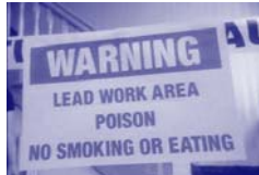
Post warning signs to keep residents out of the work area.
