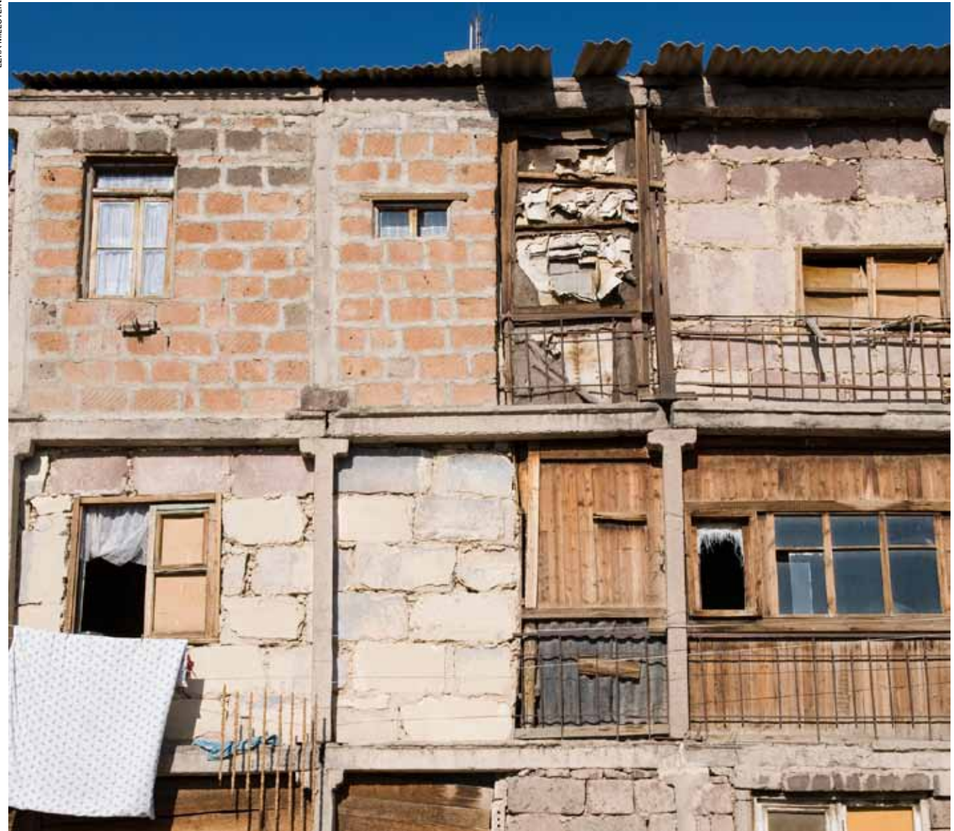
A crumbling Soviet-era apartment building.
