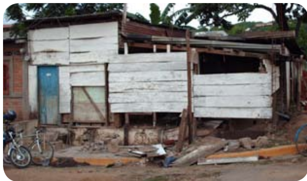
A home in a Nicaraguan community before receiving construction assistance
