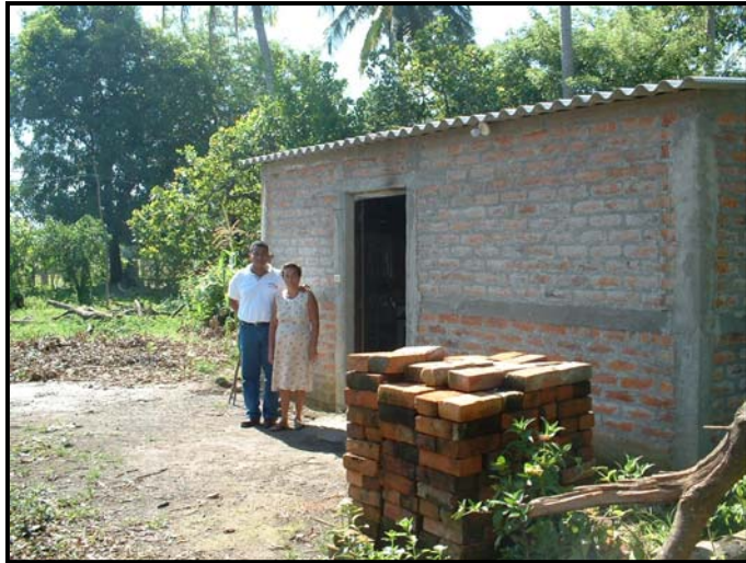
Alba Magda Miranda, an Integral client, near Zacatelocua, El Salvador, in front of her new 48m2 home. She built the house with a $1,740 loan from Integral, plus $750 of her savings. Note the horizontal cement reinforcement to protect against earthquakes.
