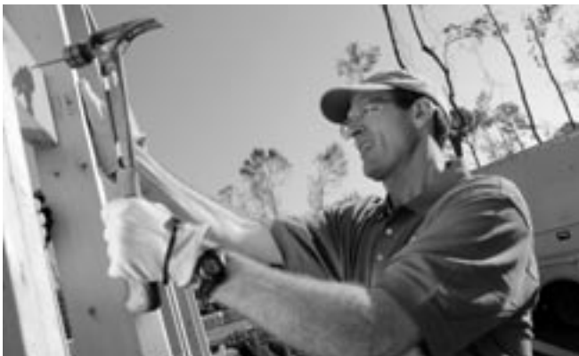
Jonathan Reckford, CEO of Habitat for Humanity International, works on a house in Covington, Louisiana, an area that was devastated by Hurricane Katrina.
