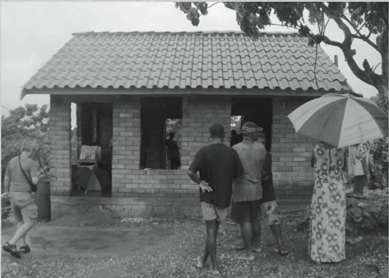
HFH Vanuatu uses tiles made out of cement rather than metal. These strong, hurricane-proof tiles can be made on site.
