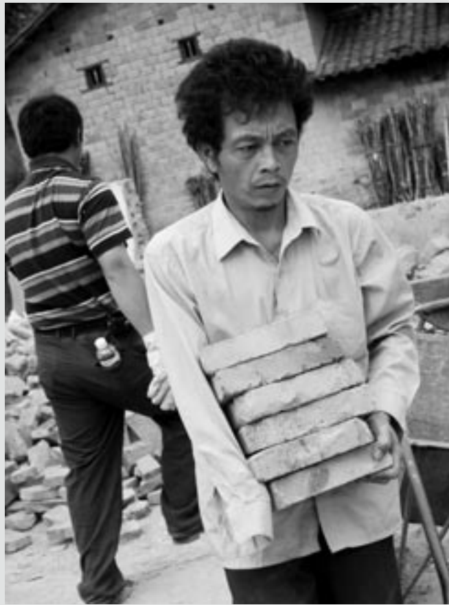
A disabled homepartner from Changliu village, Guangdong, China, contributes sweat equity for the construction of his house.
