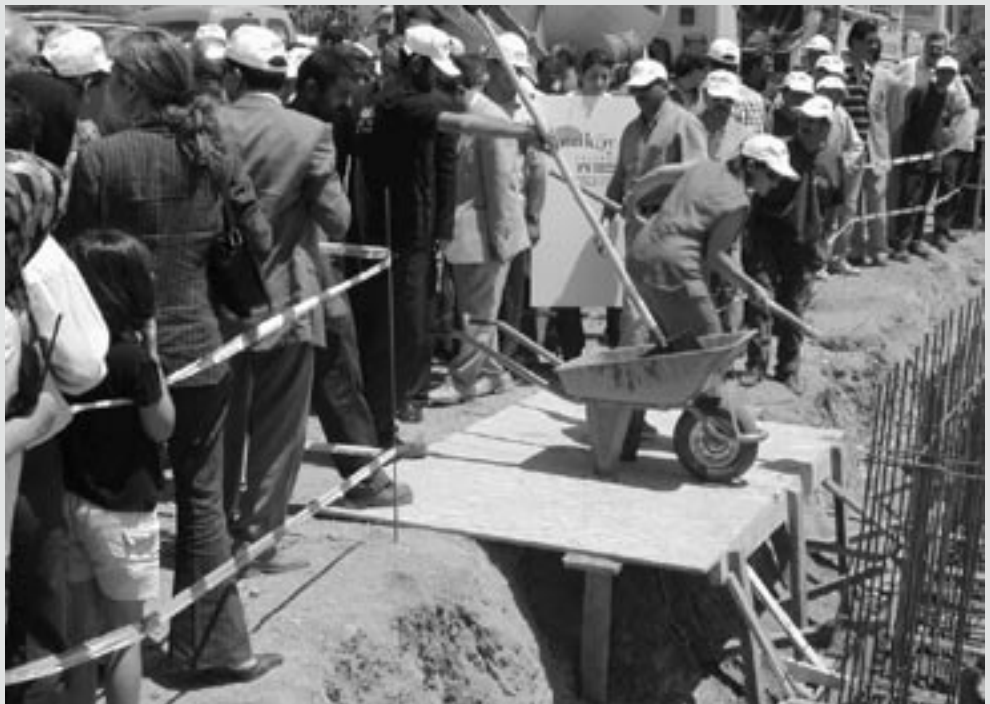
Groundbreaking at Beriköy.
