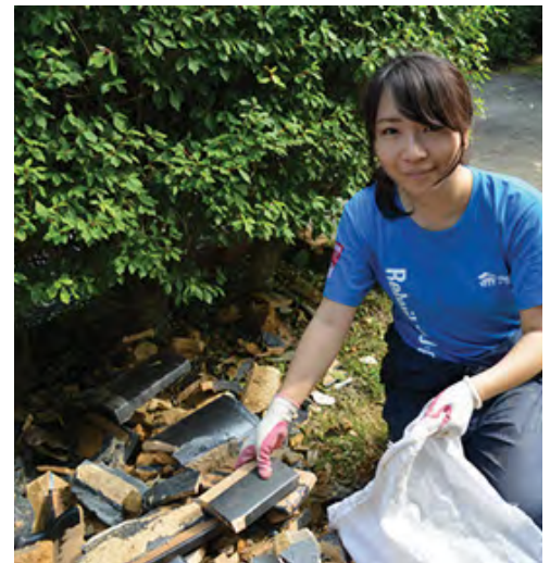
Sumire Takemura joined a Habitat volunteer team to clear debris, among other work, in earthquake-affected Kumamoto following the April 2016 earthquakes.
