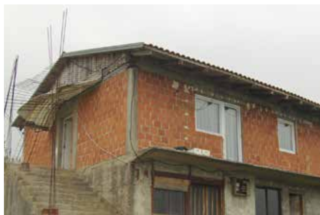
This house is in the process of being improved.
