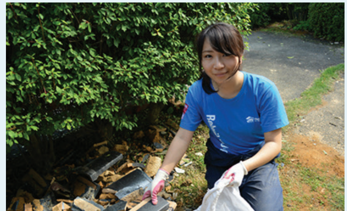
Sumire Takemura joined a Habitat volunteer team to clear debris, among other work, in earthquake-affected Kumamoto following the April 2016 earthquakes.
