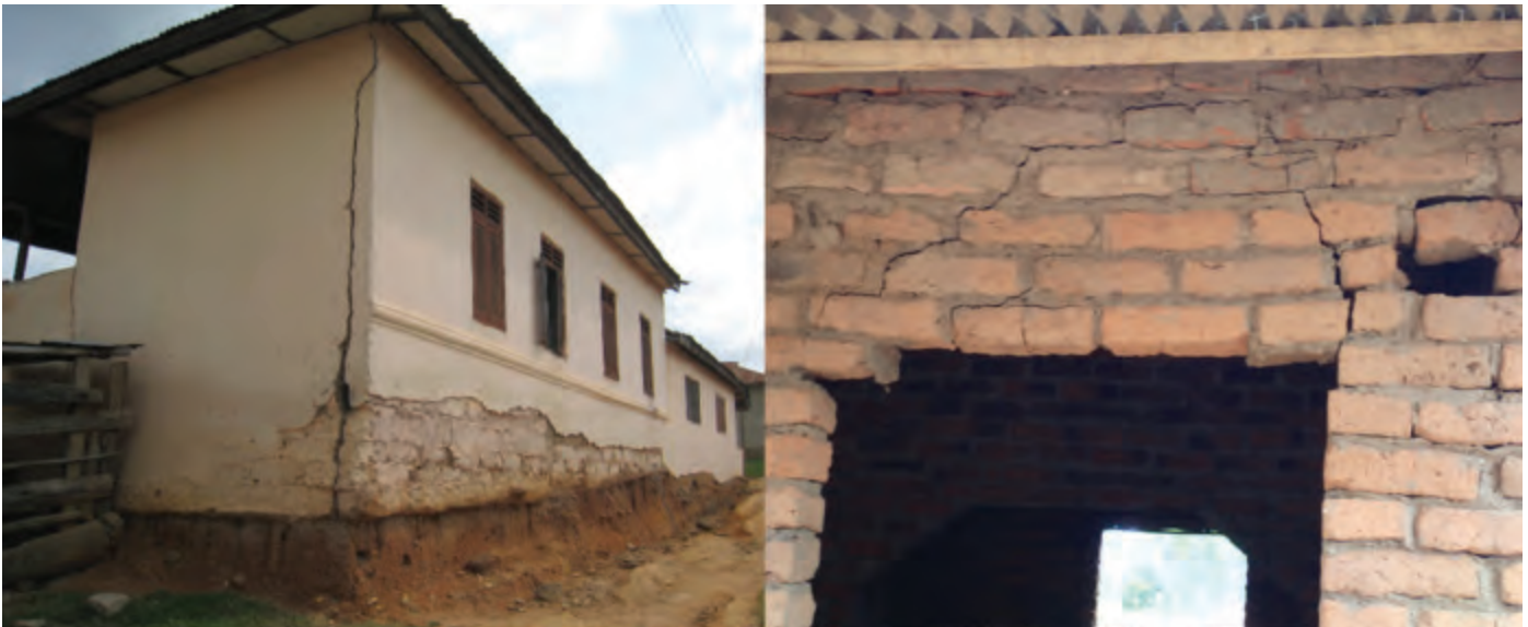
Foundation weakened from erosion; no header or lintel in window.
