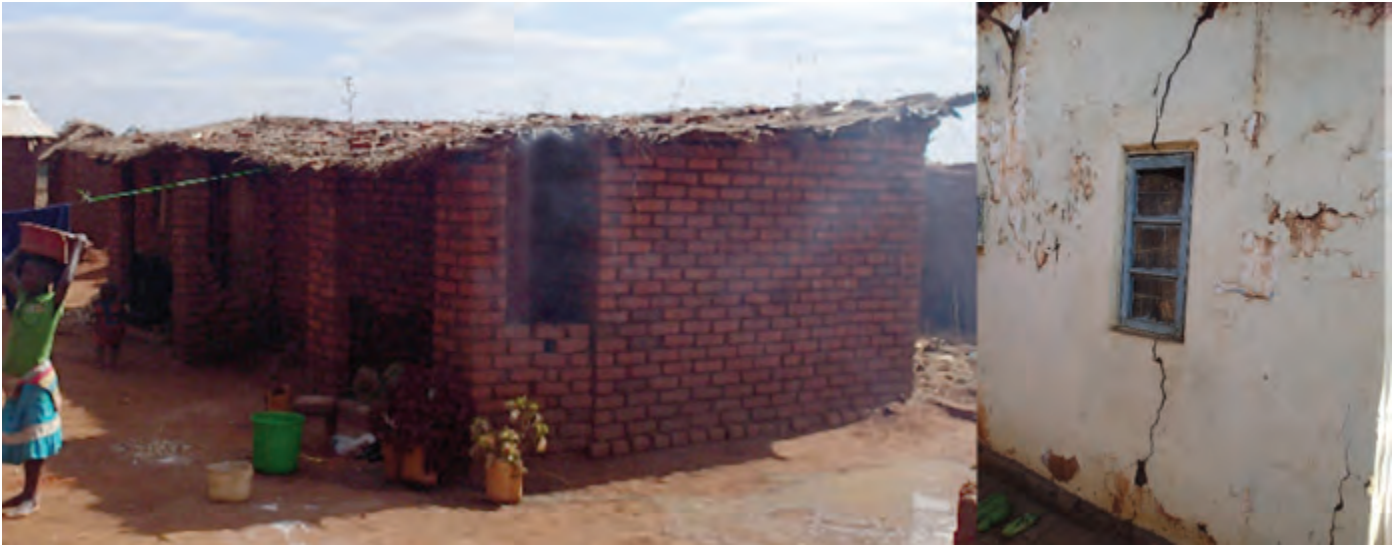
Poor roofing material and ventilation; cracks caused by poor mix.
