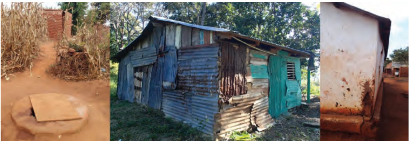
Sanitation too close to water; poor materials; poor construction leading to a failing wall.
