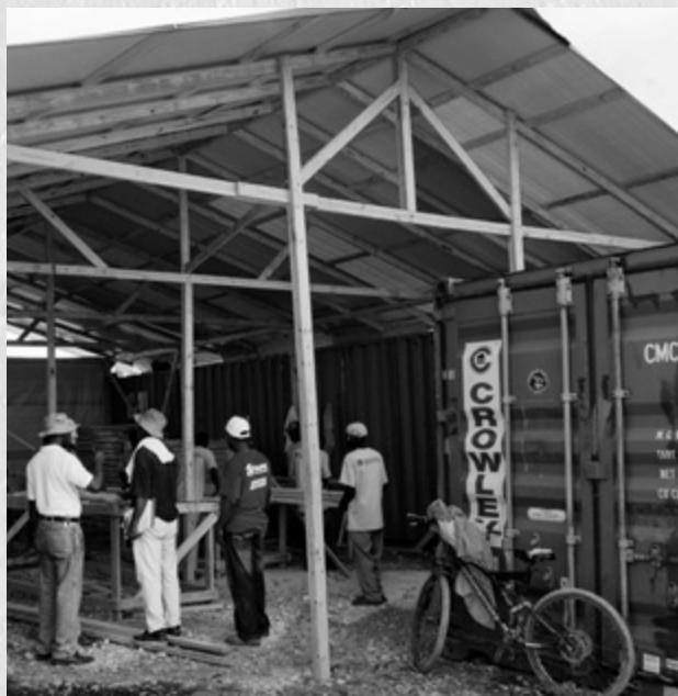
The Habitat Resource Center in Léogâne, Haiti.
