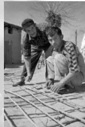
Local community workers in Tajikistan are assembling grids from mulberry branches.
