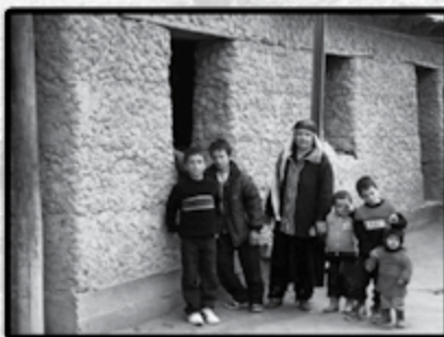
A partner family stands proudly in front of their newly reinforced home.
