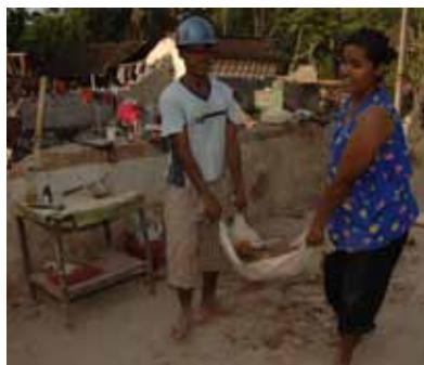
Family clears foundation to build temporary shelter.
