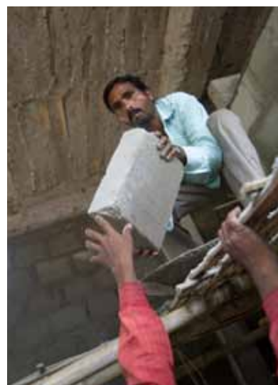
Top: Community center under construction.
