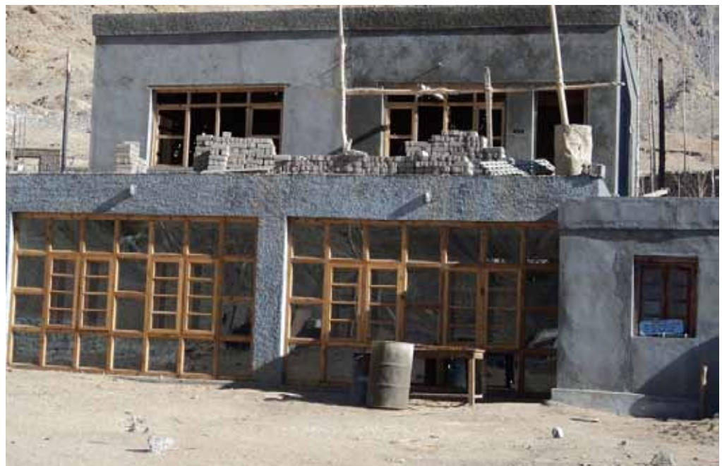
Right: House near completion.
