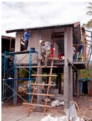
A new home built on stilts to mitigate against future flooding in Lopburi.
