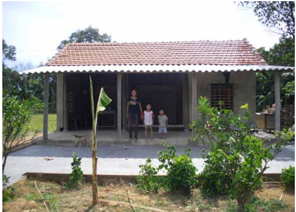
Right: Tran Thi Lai's new home.
