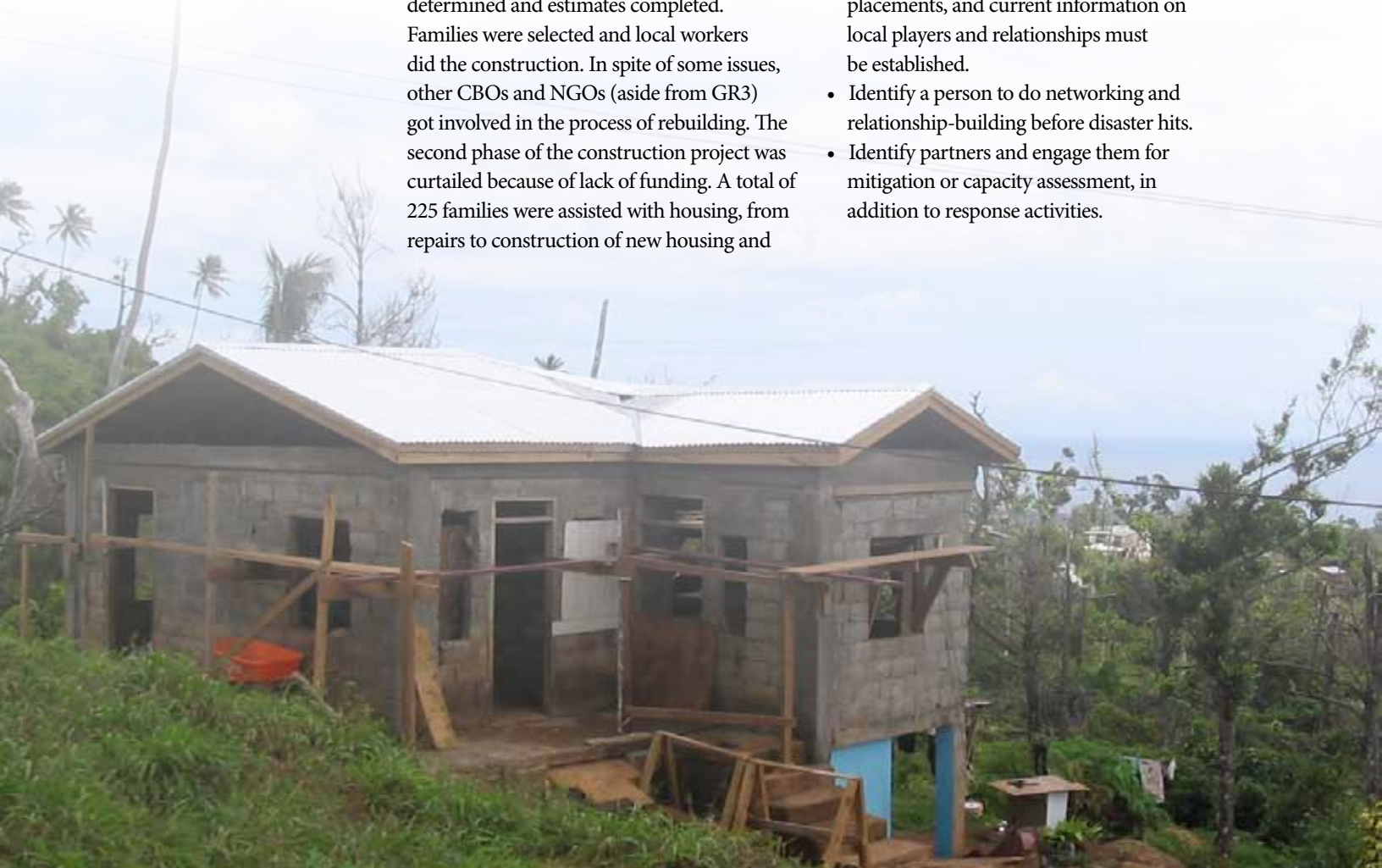
House under repair in St. Andrew.
