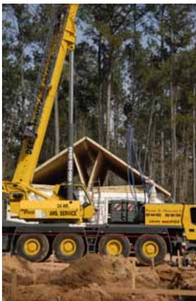
Modular houses are built in a factory and transported to a lot. A crane places the modular on its permanent foundation.
