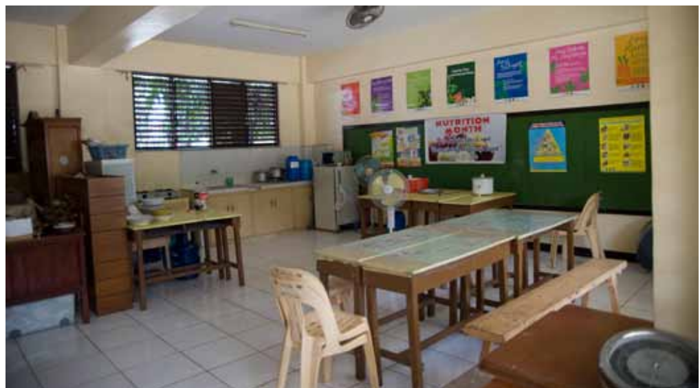
A restored classroom in Malanday Elementary School.
