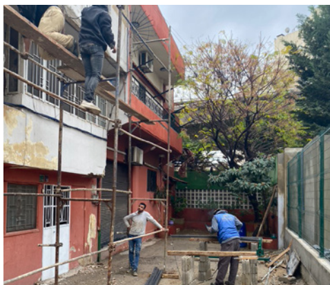
Lebanon: A multistory building's facade is repaired after damage caused by the Beirut Port explosion.
