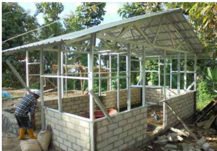
INDONESIA: Core housing under construction. The skeleton follows the recommendations for safe construction, both in the concrete blocks' plinth and in the lightweight steel structure for walls and roofing.
