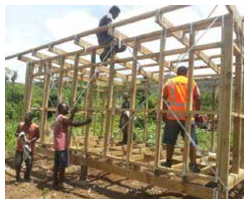
FIJI: Wooden housing under construction as part of the communities' safe shelter training program, observing the recommendations to ensure resistance, such as treated wood of adequate sections and metallic hardware (diagonals and hurricane straps).
