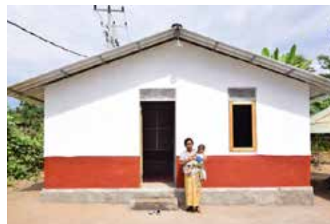
INDONESIA: Completed core housing. The interior floor is elevated with respect to the exterior to prevent the entry of torrential rainwater.
