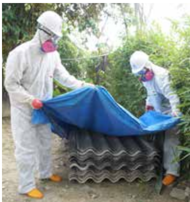
VIETNAM: Teams properly and safely dismantle unhealthy asbestos sheeting roofs.
