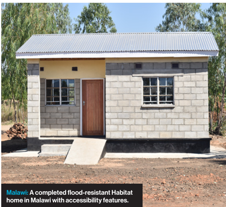
Malawi: Habitat Malawi constructed homes with an elevated foundation.
