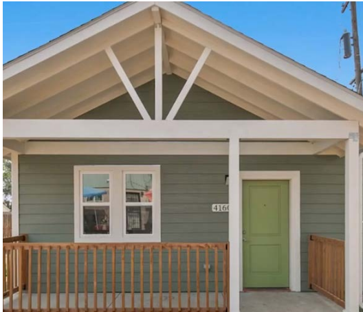
Source: Habitat for Humanity
