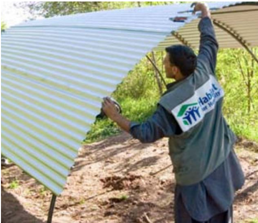
Source: Habitat for Humanity
