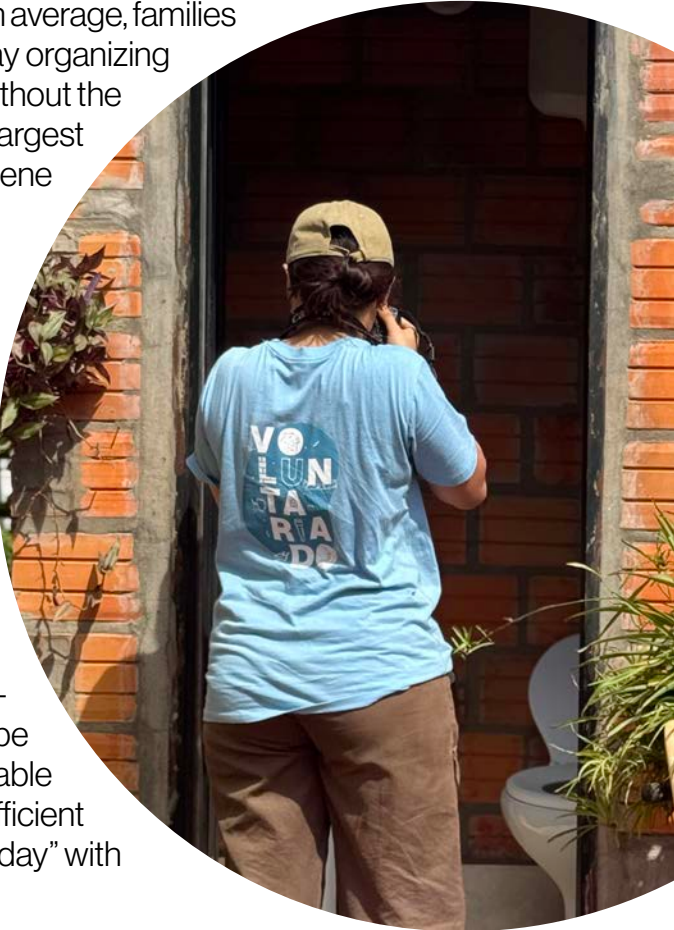
Sabrina photographs the bathroom installation.
