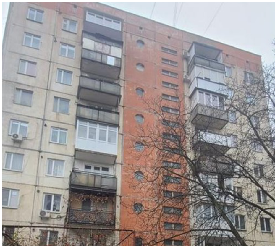
Picture 5. Reinforced concrete structures building.
