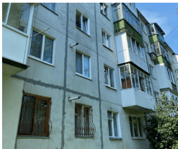
Picture 4. Panel house building.
