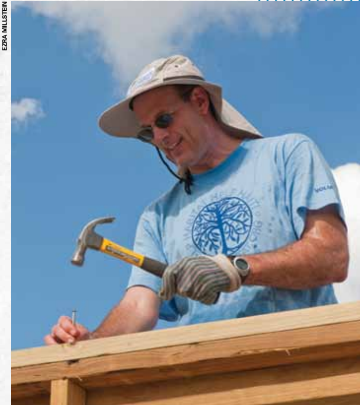
Habitat CEO Jonathan Reckford pitches in to help build one of 100 houses at the 28th Jimmy & Rosalynn Carter Work Project in Léogâne, Haiti, in November 2011. An additional 100 houses will be built when the Carter Project returns to Haiti in November 2012.
