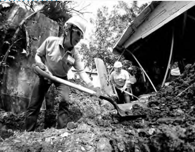
Elizabeth Crossman, Habitat for Humanity International board chair, hones her building skills on a Habitat for Humanity build site in the Dominican Republic in November 2011.
