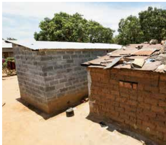
The structure on the left is a Habitat home built with sturdy cement block. The one on the right is made of unsafe porous mud brick.
