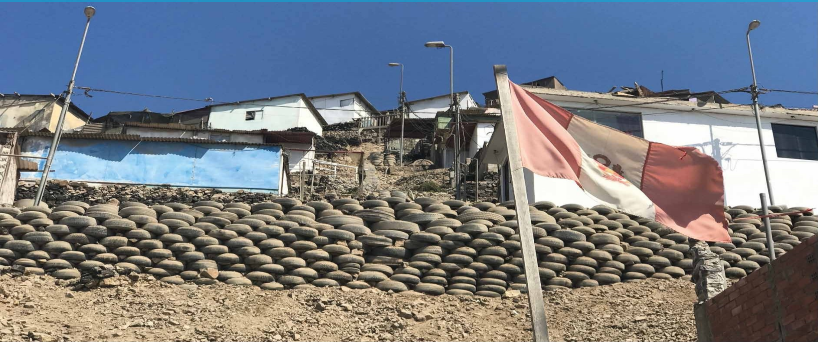
2019 - Chorrillos, Lima. Peru: Due to lack of information and professional advice, it is very common to see that houses in peripheral areas of the city use tires as part of their foundations. Photography: Fernando Ocampo
