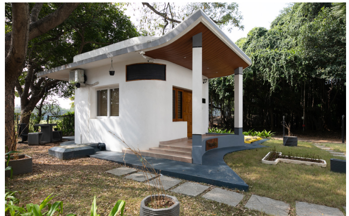
With support from The Terwilliger Center, Tvasta Manufacturing Solutions built what is believed to be the first 3D-printed home in India.
