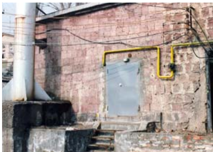
“Jrashat 92” boiler house
