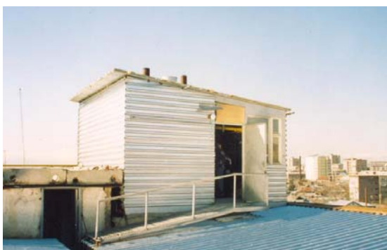
The top-roof boiler house of the building #106 on P. Sevak st.
