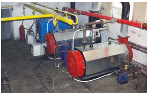
Boilers installed at "Jrashat 92" boiler house
