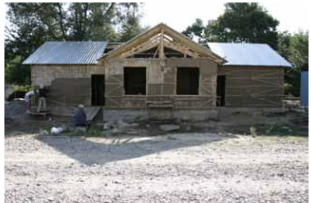
A cane-reed house under construction.
